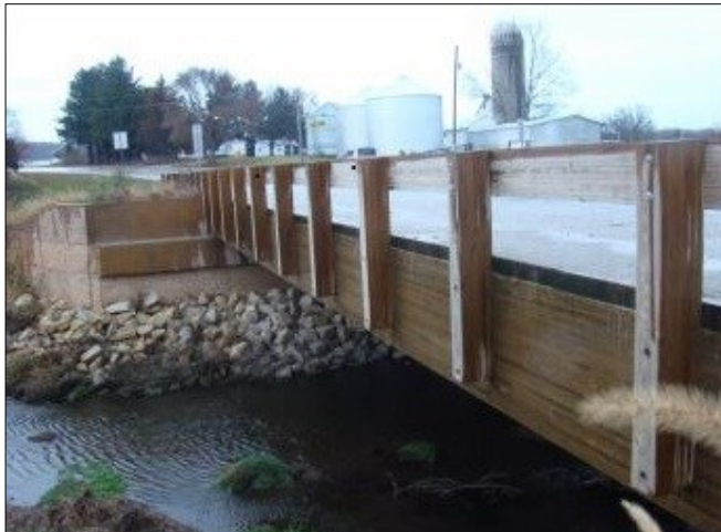
Figure 1. Glulam girder timber bridge in Buchanan County, Iowa. (Photo credit: Zach Carnahan)
