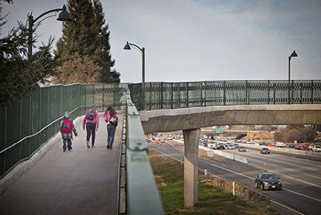
Pedestrian bridges over freeways are safe and convenient ways to encourage active transportation. Photos Courtesy of Headquarters Photography
